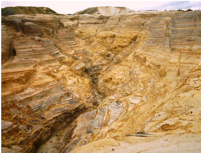
Eroding tailings dam near Smeaton.
